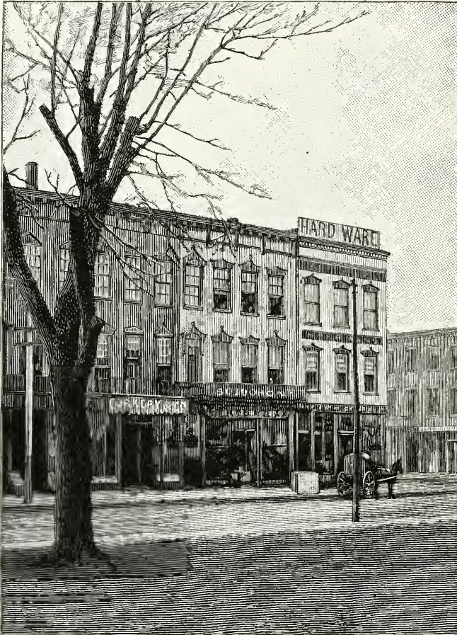
LINCOLN & HERNDON'S OFFICE IN THE THIRD BUILDING FROM THE CORNER.
